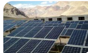
Leh and Kargil Solar Power Projects, India
